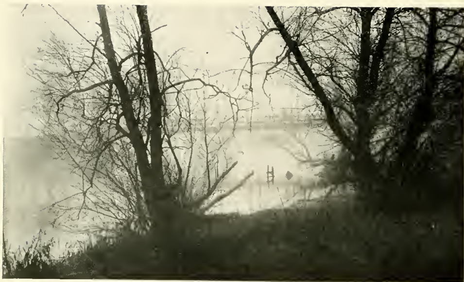
BRIDGE ACROSS DES MOINES RIVER, WINDOM.
